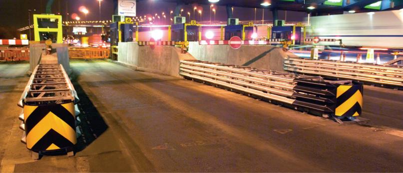
Trinity Highway Products, LLC manufactures the EURO-TRACC™ with galvanized all-steel construction that reduces concern of product deterioration from the sun's ultra-violet rays and extends service life with minimal maintenance by end users. Interchangeable components facilitate swift and inexpensive repairs for highway agencies and departments of transportation.
