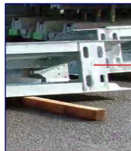
Ground Fixing Point
