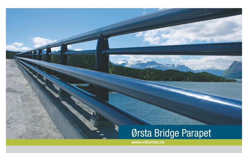
Orsta Bridge Parapet has been full scale tested in accordance with NS-EN 1317 in containment class H2 and working width W2.
